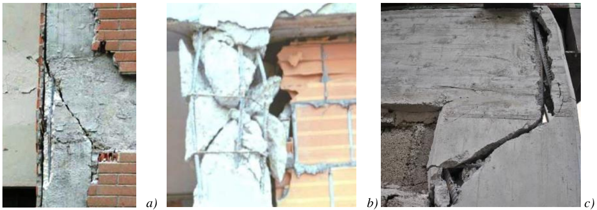
Figure 2. Local failures of RC frames due to the interaction with infills: a) Failure of a joint; b) Failure of a column end; c) Failure of column and joint.
