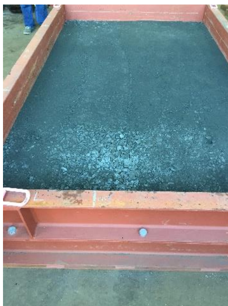
Figure 6. 400mm height of subballast
