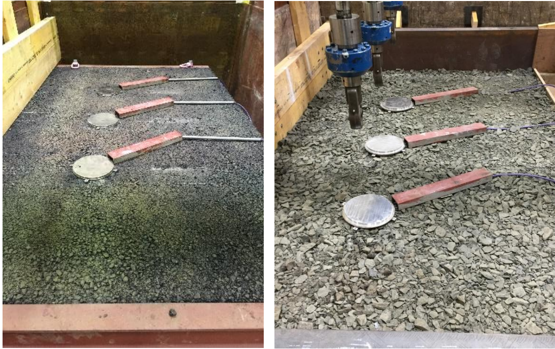
Figure 9. Placement of pressure cell plate in asphalt-ballast track (left) and ballasted track (right)
