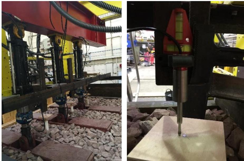
Figure 11. Installation of actuators (left) and Installation of LVDTs(right)
