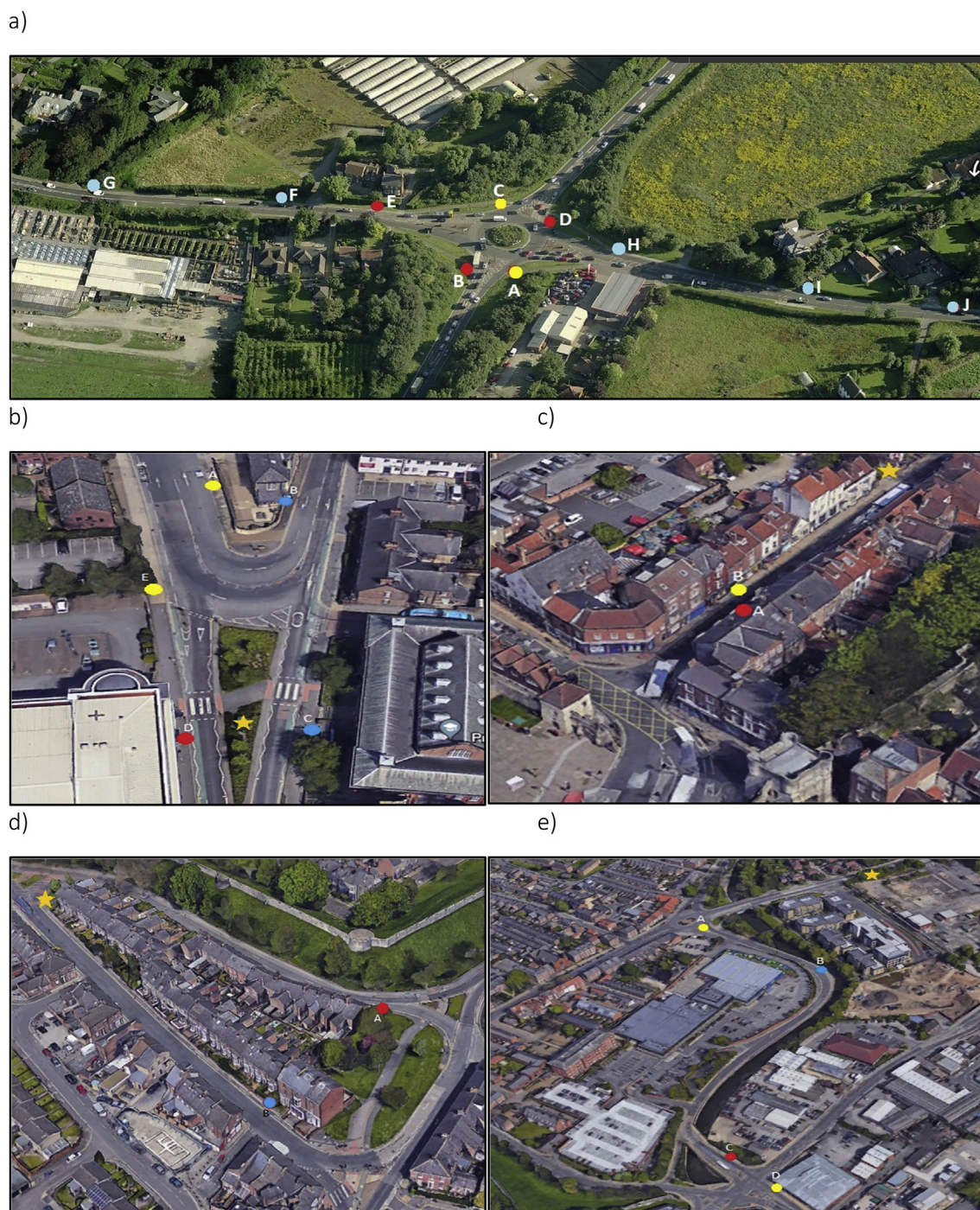
Fig. 2. Aerial photographs from due South (Microsoft, 2017) of a) Ring road (A59/A1237) roundabout, b) Fishergate one-way system, c) Gillygate/Bootham junction, d) Nunnery Lane/Prices Lane one-way system and e) Foss Bank. Labelled points (A–J) of the diffusion tubes at each location where traffic predominantly accelerates (yellow), queues (red) and cruises/slows (blue) during peak traffic times. In-situ monitor locations (yellow star). (For interpretation of the references to colour in this figure legend, the reader is referred to the Web version of this article.)
