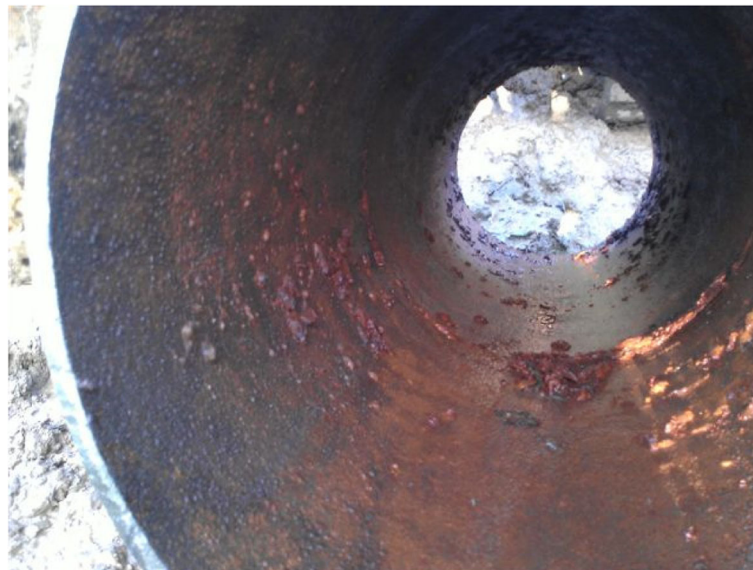
Fig. 1 The interior of a ductile iron main that was drained down to repair a leak. Note the thin (particulate) material coating the complete pipe wall, as well as larger more stable corrosion tubercles
