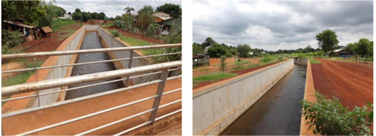
Figure 24. The water of the Tacuara stream confined into a concrete channel
