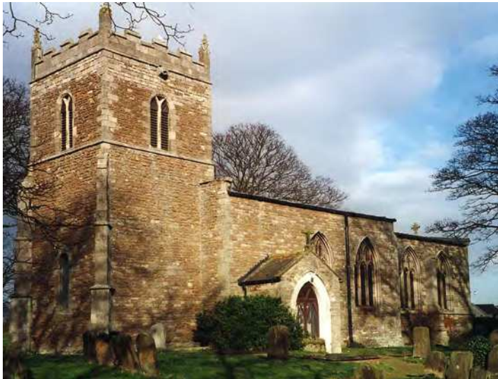
FIGURE 1-7 The church of St Etheldreda, West Halton, from the south west.
