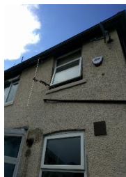
Fig. 15. VHF TX antenna located at the first floor window of dwelling.
