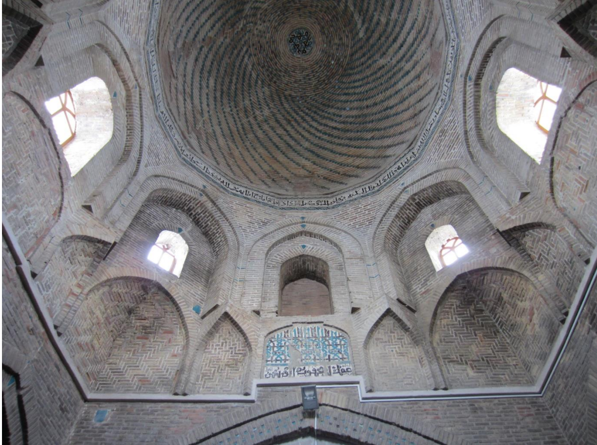
Fig. 12 – Malatya Great Mosque (645/1247); large structural brick muqarnas cells in maqṣūra dome squinches © R. McClary
