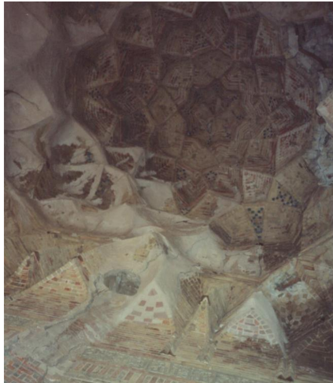
Figure 17 Upper section of the muqarnas cell ceiling © Katie Marsh
