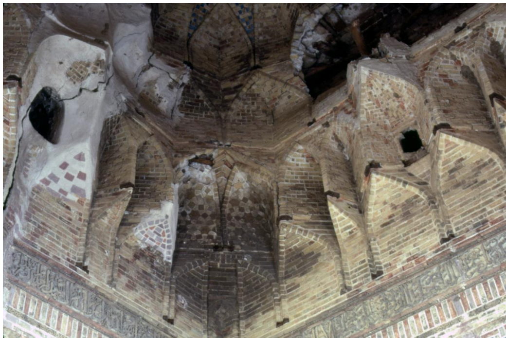
Figure 18 Lower portion of the muqarnas cell ceiling © Yasser Tabbaa Archive, Aga Khan Documentation Center at MIT
