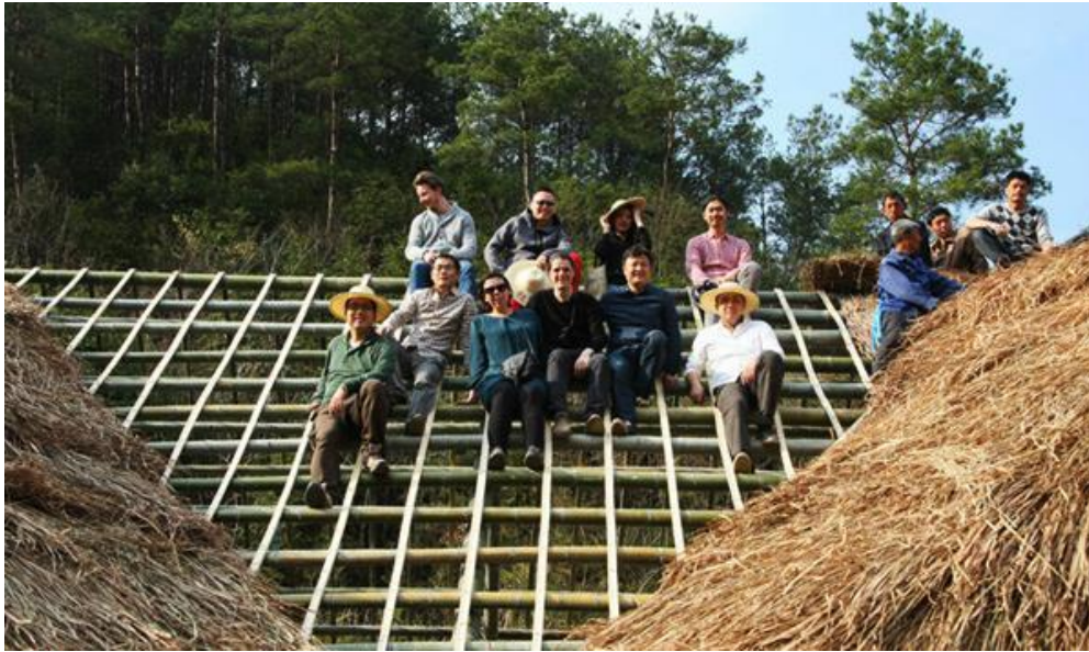
Figure 7. Group photo of roof builders. Source: Sun Commune
