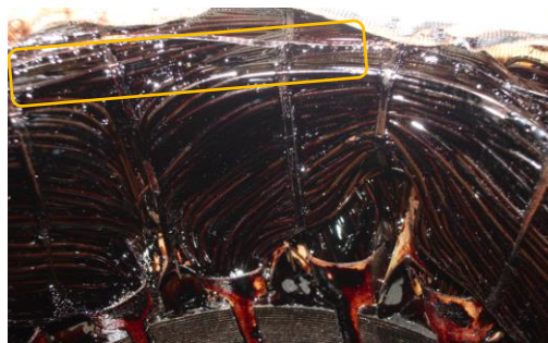
Fig. 10 Sample 3 End-Windings After Failure. Phase-phase overlap in the EW region is highlighted
