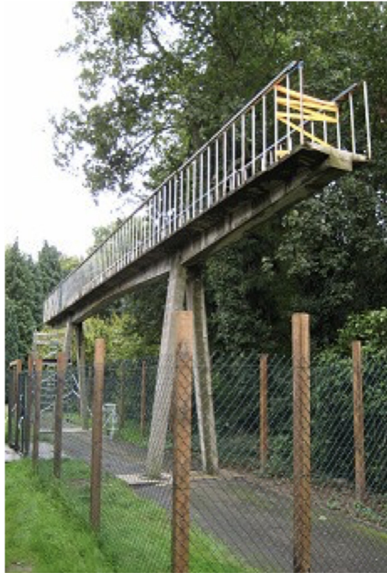
Fig. 11. The photo of the NPL Bridge in situ.
