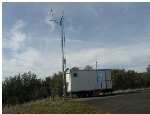
Figure 21: Photograph of the Paradise Airport, USA, air quality remote monitoring station (Wey et al. , 2006).
