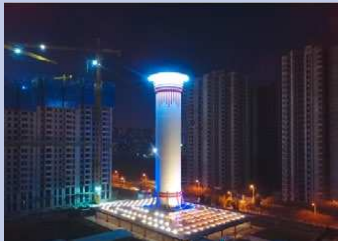
Figure B A night-view of the 1st generation SALSCS built in Xi'an, Shaanxi Province (completed July 2016)
