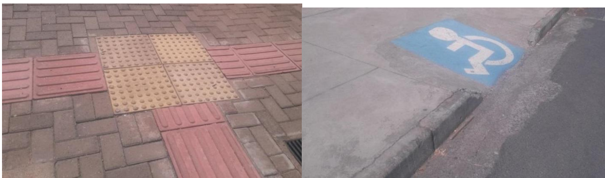
Figure 65 and Figure 66 - CEU sidewalks paving
