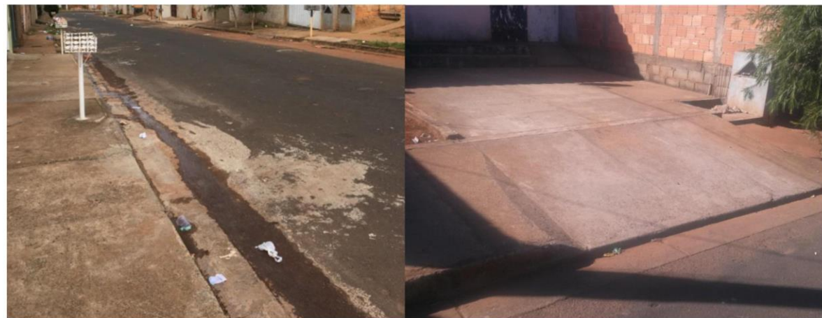
STREETS AND SIDEWALKS WITH NO PROPER SLOPE
