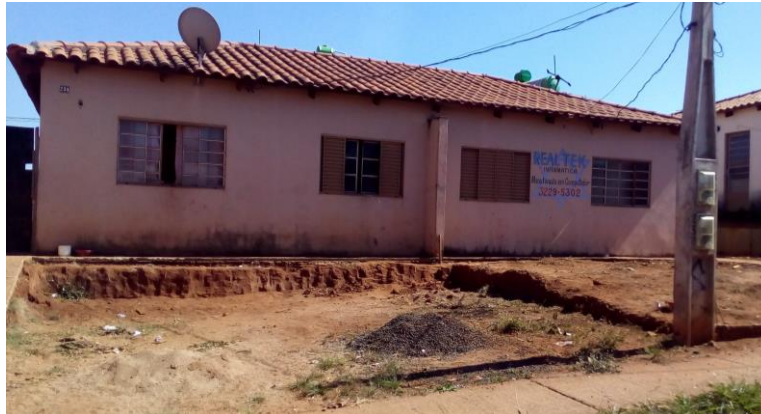
Figure 280 - Frontal facade of 2 of the houses whose backs are shared.
