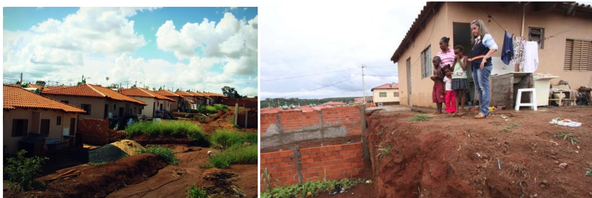
Figure 214 - Houses location and landslide accident
