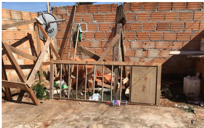
Figure 261 - Residues placed behind a house.
