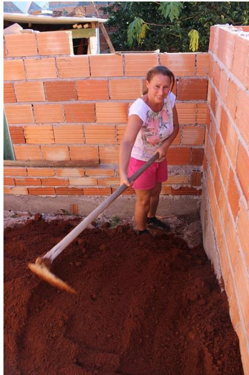
Figure 274 - Dweller refurbishing her own house.
