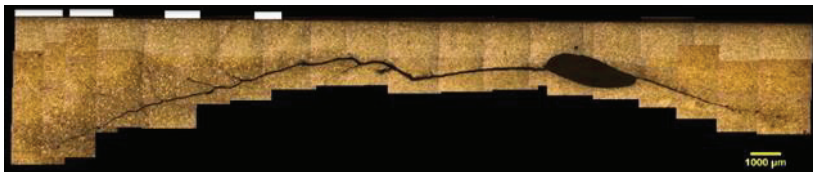
Fig. 2. Example of massive void morphology below the running band in a longitudinal cross section from a high speed mixed traffic line. The central portion of the defect lies approximately 2 mm below the rail surface. Incline crack initiated from the left and right side of the void. The white marker above the rail surface indicates the location of a patch of white etching layer with a thickness ranging between 20 to 250 μm.
