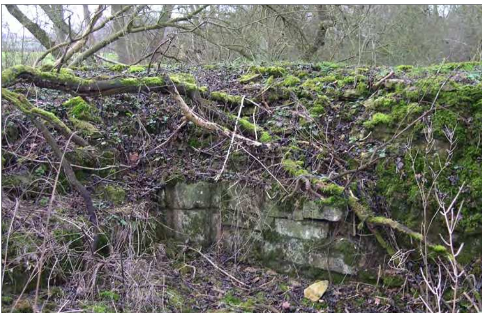
(c) Torpel Lodge remains: the interior southwest corner contains the sole remaining section of ashlar facing. The workmanship is of high quality and the courses vary between 8 and 11cm in height. The shaft was presumably the springer for rib-vaulting, forming the ceiling of the ground floor.
