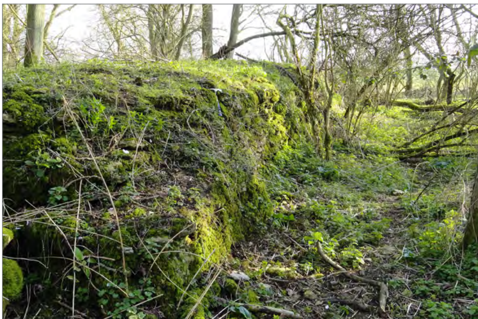
(b): Torpel Lodge remains: northwest corner, looking south externally. The coursed rubble walling would have been originally faced with limestone ashlar. The corner in the foreground appears to have carried pilaster buttresses.
