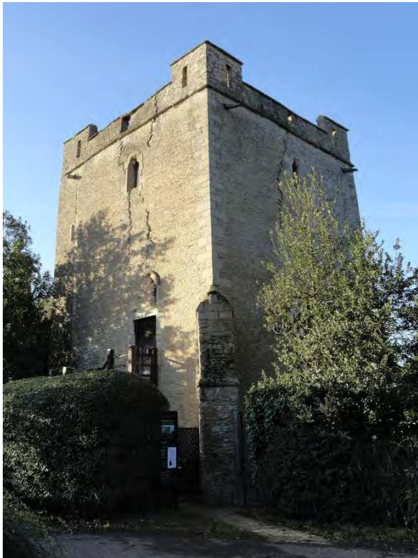
Figure 44: Longthorpe Tower. This gives a general impression of the original form that Torpel Lodge may have taken.
