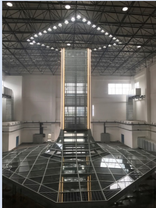
Figure C The 2 nd generation SALSCS built in Yancheng Science Park, Jiangsu Province (completed September 2017)
