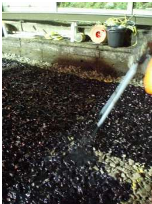
Figure 10: Pouring of the polymer at the site
