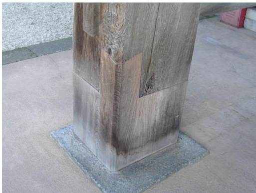
Figure 7 A new timber component was used to partially replace a rotten column with traditional carpentry
