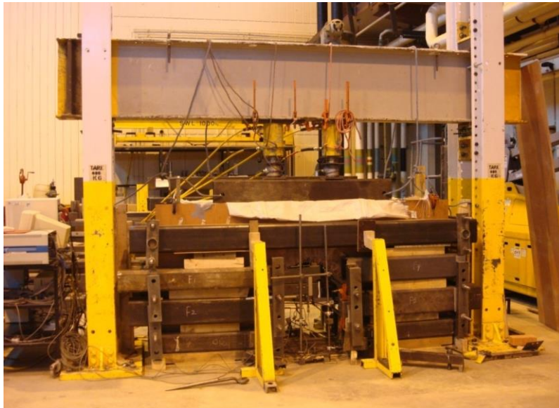
Fig 2. Loading system installation for uniform load (Chen, 2014)
