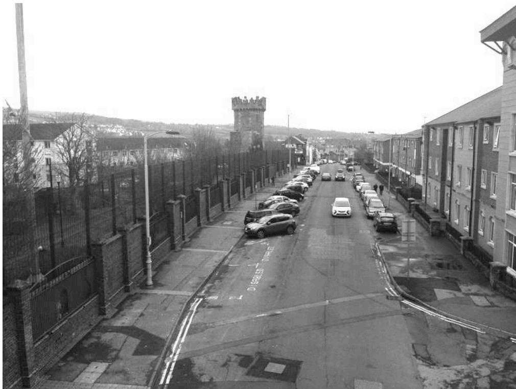
Fig. 5. Peace wall running alongside Bishop Street and the Fountain Estate
