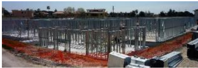
Figure 4: Cold formed steel low rise building, (Fiorino, et al [6]).
