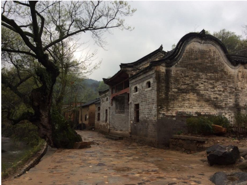
5 Ancestral Hall of surname Zhang of Xihe Village, oriented north-south and located at the starting point of market street, is just confronting the site for the new community centre on the opposite side of the river. Spring 2015
