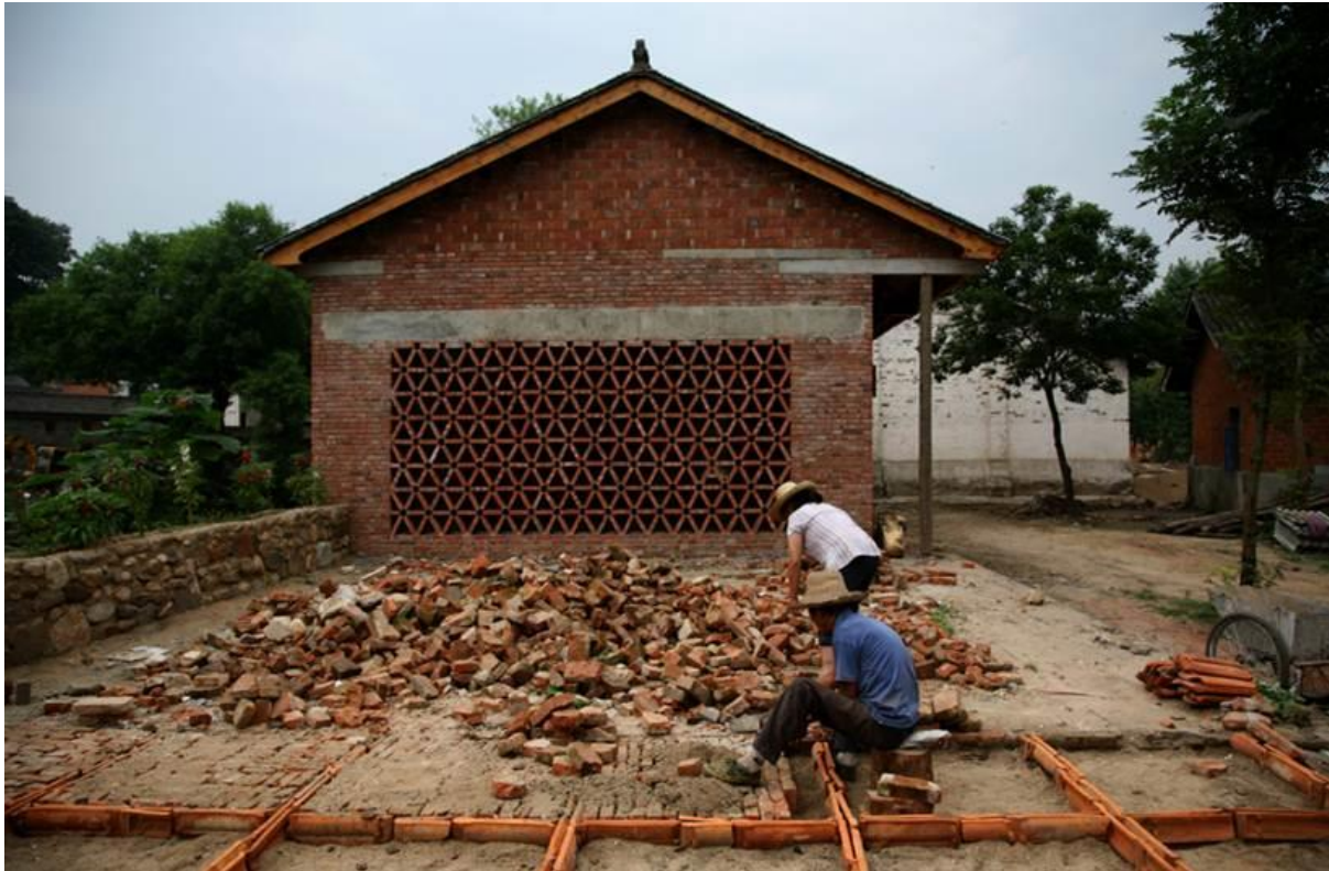
16 Collective construction process on site. Summer 2014
