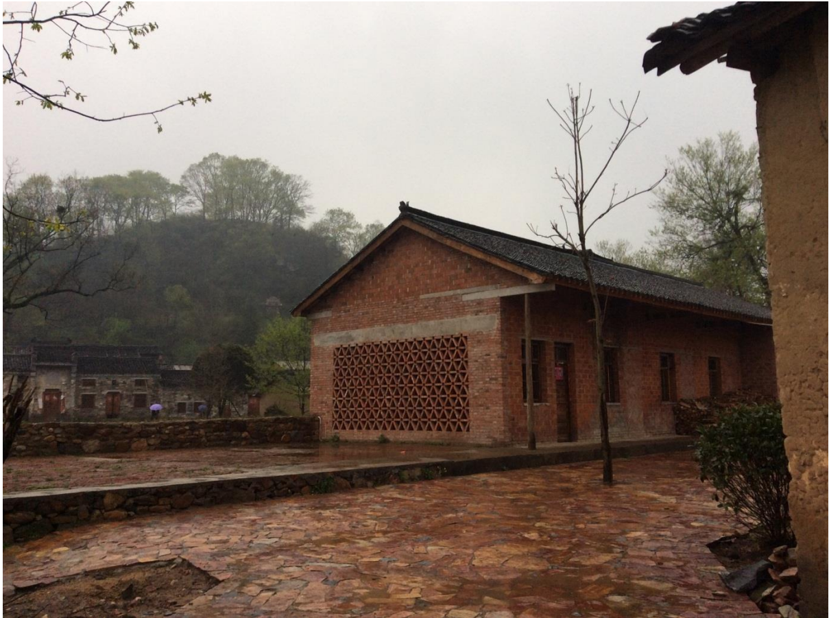
13 A new canteen for the village was transformed from an abandoned building, with its external brick-screen-wall coproduced by the architect and users in a different way from both urban and rural normal practice. One third of the existing volume was demolished in order to leave a ritual visual corridor to assimilate Qi (energy) to the main body of village on the other side of the river. Spring 2015
