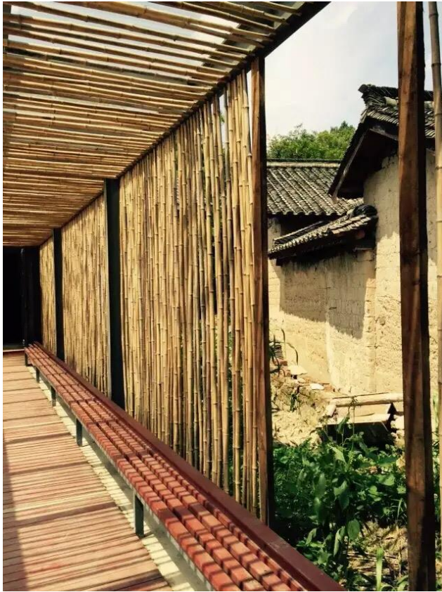
11 A light-weight corridor connects the community hall and the mini-museum, and provides a linear space under the eave to enclose the public square in between. Summer 2015
