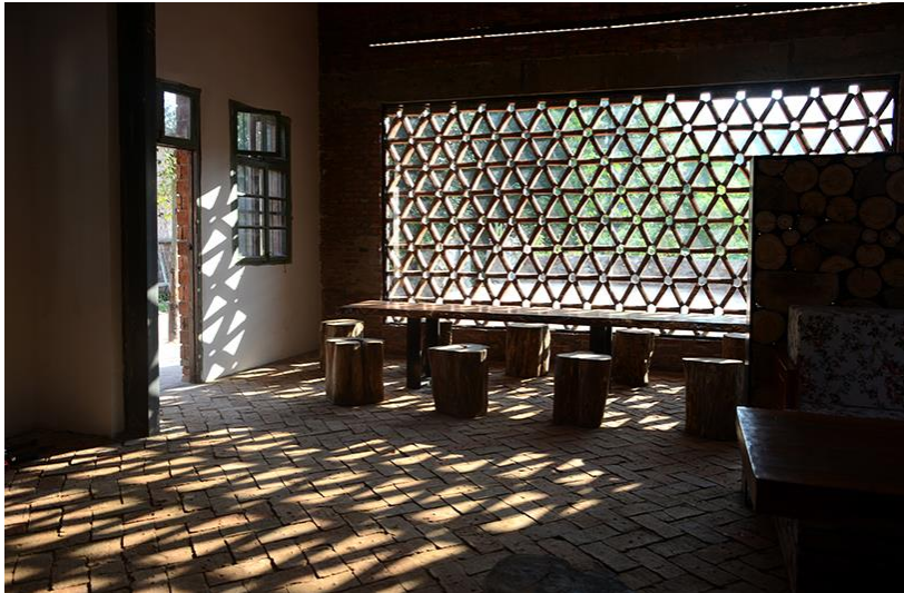
17 Interior of canteen after completion. Autumn 2014 A perforated brick-screen wall provides sunshades and changing patterns of light and shadow.
