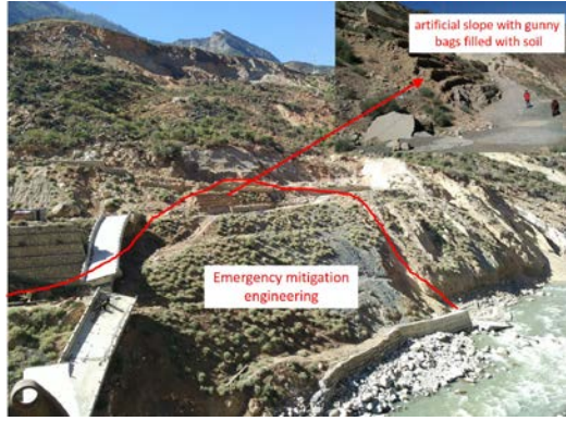
Fig. 15. Artificial slope (photograph taken 12 th December 2015).
