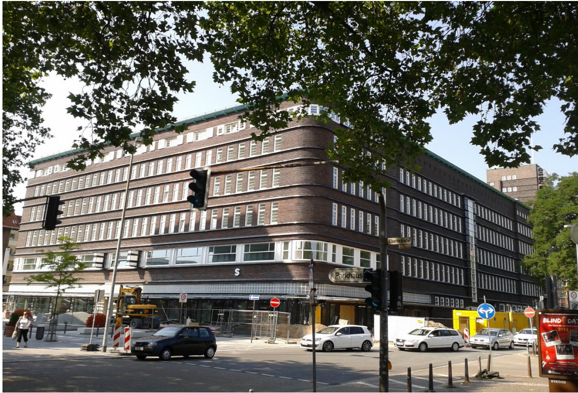
Figure 3: Hans-Sachs-Haus shortly before it was reopened (photograph taken in July 2013)
