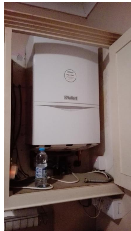
Figure 2. A modern water heating system installed in a typical UK household (the authors house). It shows very little evidence that fossil fuel is being burned inside this metal box which itself is hidden away in a cupboard.
