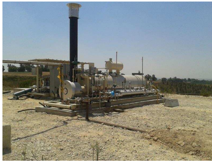
Figure 18. The heat exchanger.
