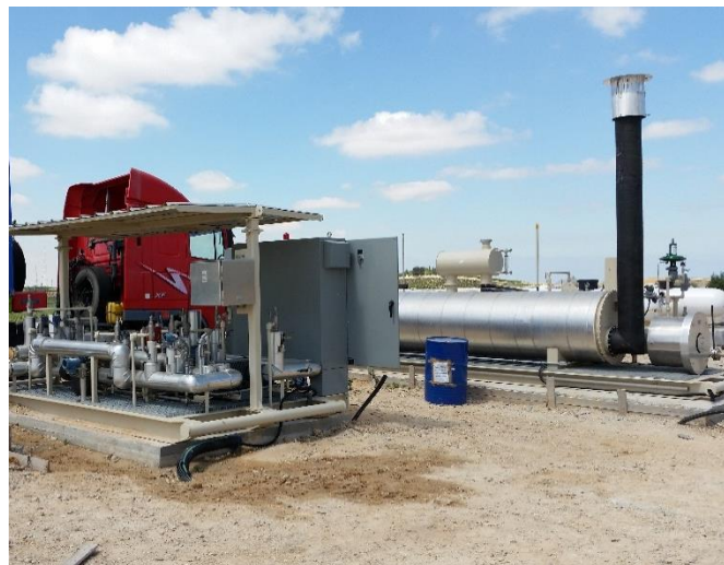
Figure 19. Pump skid during commissioning.
