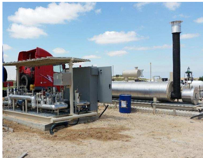
Figure 19. Pump skid during commissioning.
