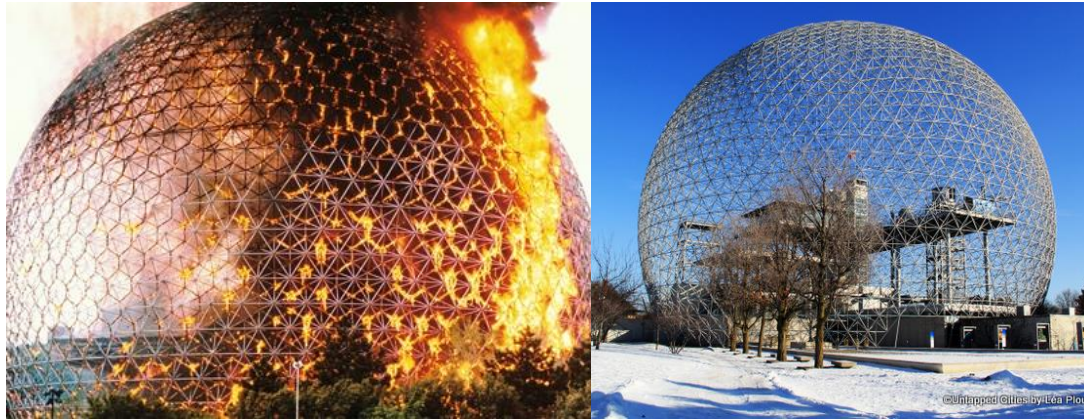
(a) During fire (b) After repair
