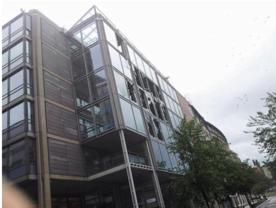
Figure 16: Window damage in a building subjected to blast loads.
