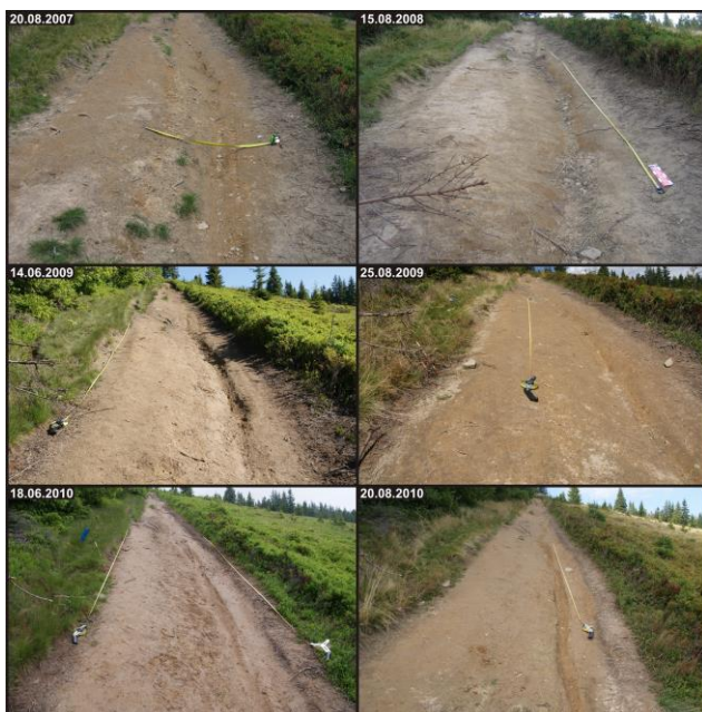
Figure 6. Case study E – an example of trail which had already been degraded before the intense rainfall event. Trail tread was uneven and wide. The extreme rainfall event caused an increase in soil erosion and the rill was deepened.
