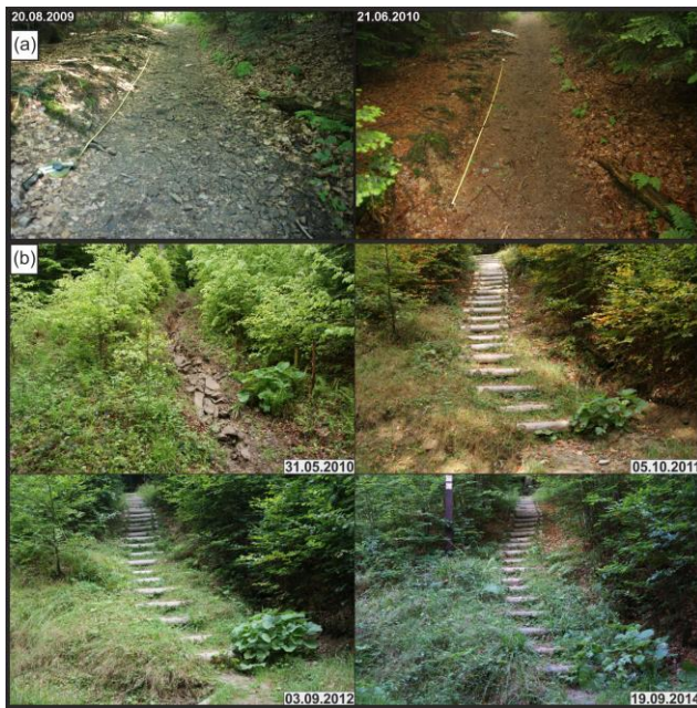
Figure 4. (a) Case study A – an example of a trail which was not damaged during the intense rainfall event which occurred in May 2010. (b) Case study B – an example of trail damage (development of an erosional rill) and the appearance of the trail after repair (scenario 2).
