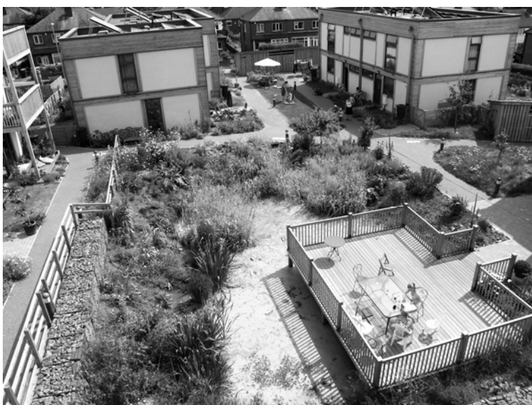
Figure 6: Central pond and homes
