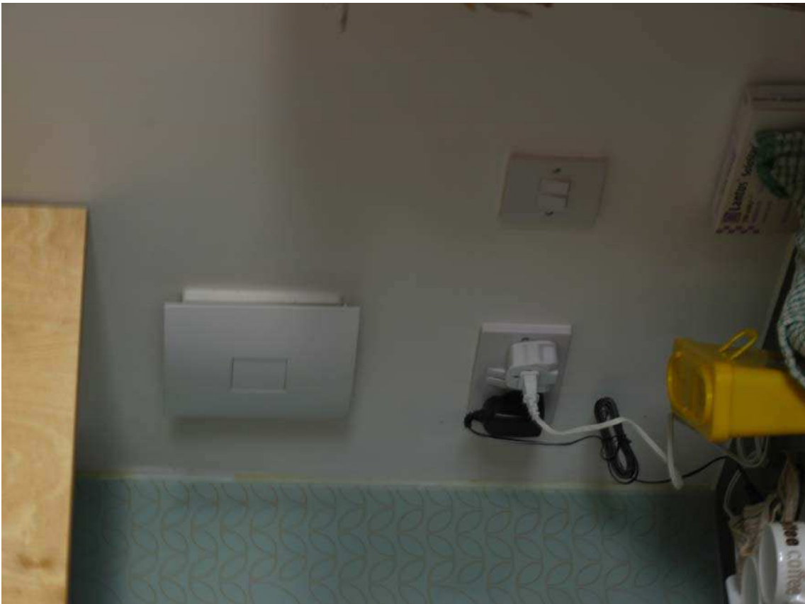
Figure 6 Decorative cover disguising MEV fan (Case B).
