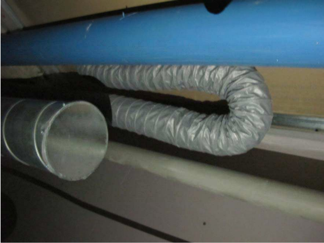
Figure 5 Too long, bent flexible ducting linking exhaust fan with the main duct (Case B)
