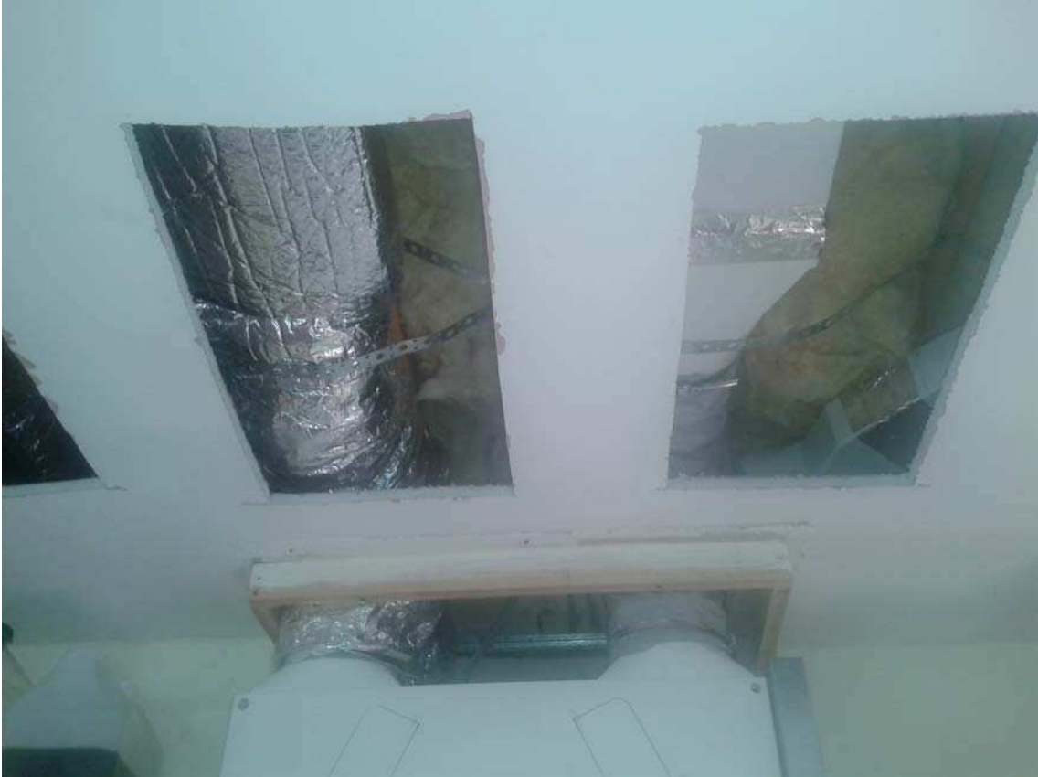
Figure 3 Ceiling taken down to insulate MVHR ducting (Case A)
