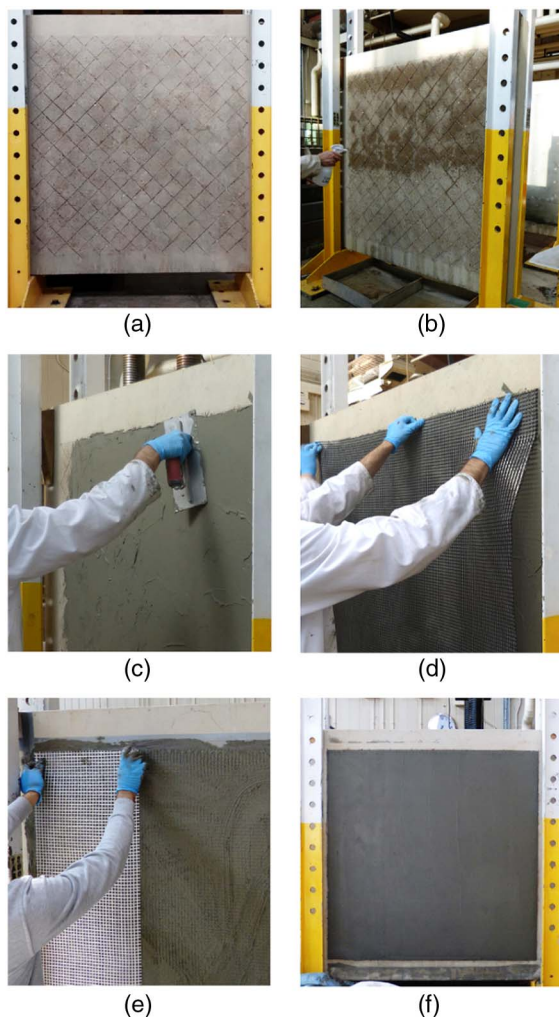
Fig. 4. TRM strengthening application steps: (a) concrete surface preparation; (b) dampening of surface to receive strengthening; (c) first mortar layer application; (d) carbon textile application; (e) patch of glass textile application; (f) final finished surface
