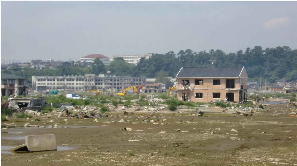
Figure 2. The tsunami reached as high as the fourth story of this apartment block overlooking the bay in Rikuzentakata, Iwate Prefecture (August 2011).
