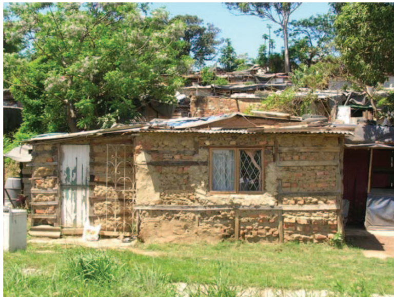
FIG. 2. Photo showing integrated burglar guards.
