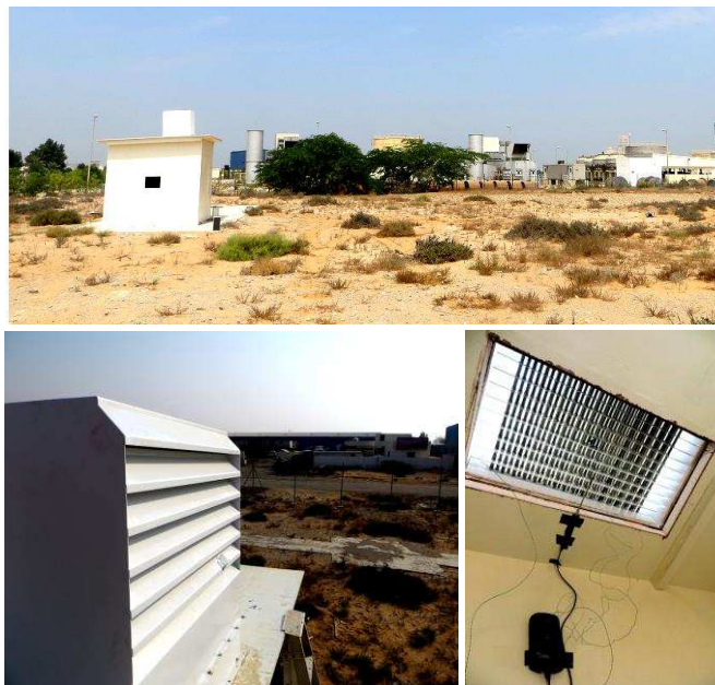
Figure 6: Test site in Ras Al-Khaimah (top) wind catcher mounted on the roof (bottom left) measurement setup (bottom right).
