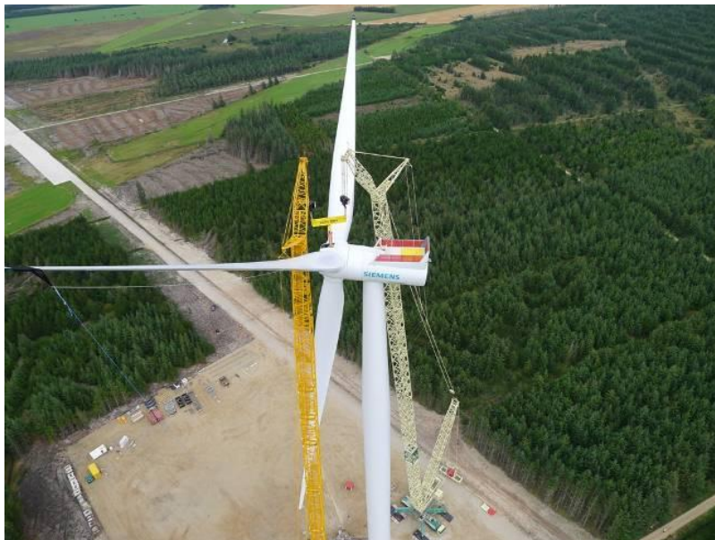
Siemens WP 6 MW DD turbine installation
