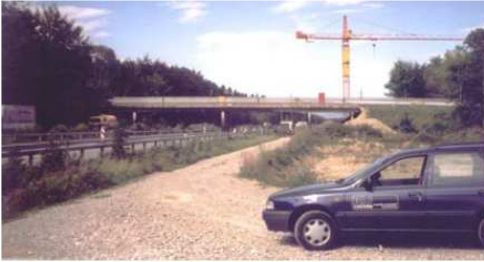
Figure 1: The Z24 bridge.
