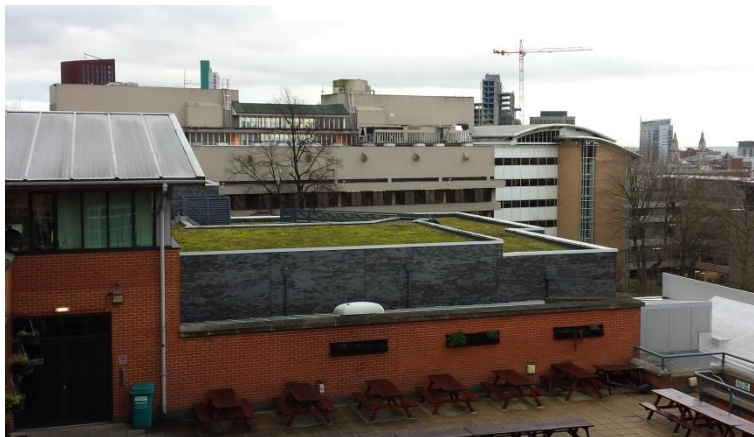
Figure 4.1.1: The extensive green roof above the University of Leeds Performing Arts building in 2007 (a.) and 2014 (b.) (McLaw Living Roofs, 2007).
