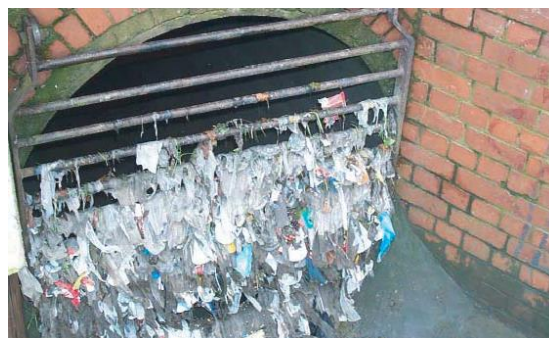
167 Figure 1.1: A combined sewer outfall in Leeds (Leeds City Council, 2004).
