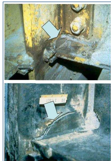
Brittle Connection Damage, 1994 Northridge
