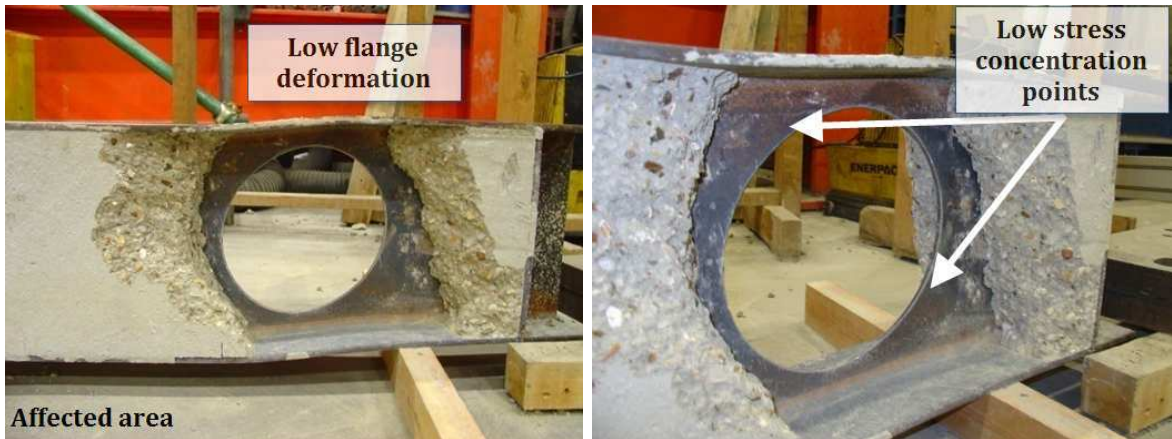
Fig. 18: Failure mode for partially encased USFB No.2 at opening after removal of the damaged concrete
