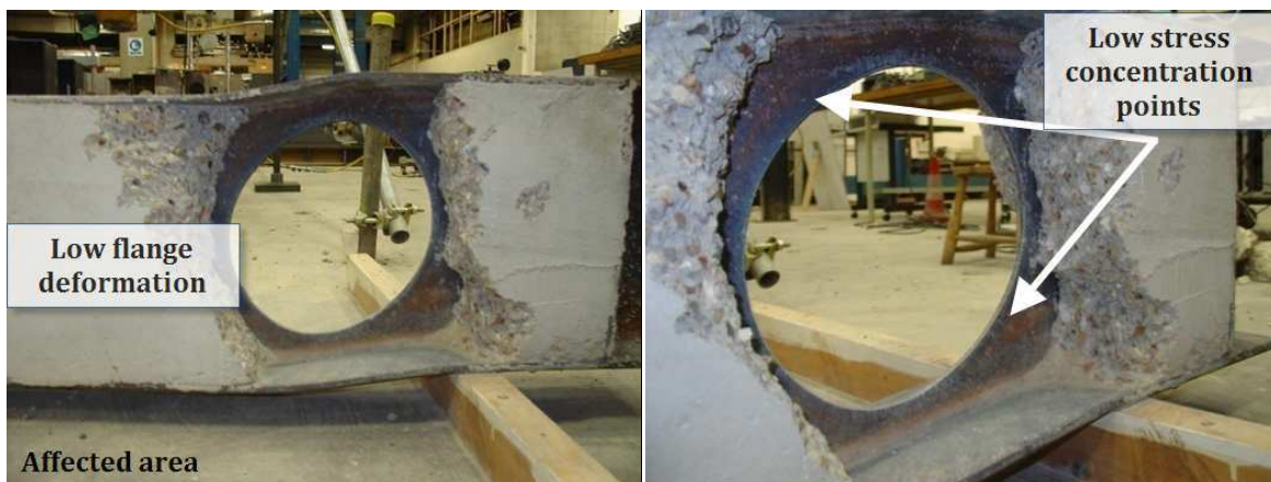
Fig. 17: Failure mode for partially encased USFB No.1 at opening after removal of the damaged concrete
