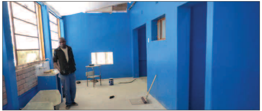
Progress on the interior.
