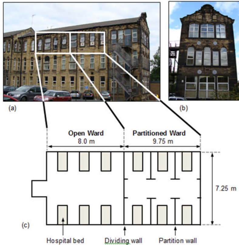
Figure 1 – (a) front view and (b) end view of the experimental facility, St. Lukes Hospital, Bradford, UK and (c) aerial schematic representation of the ward layout, featuring open and partitioned wards.
