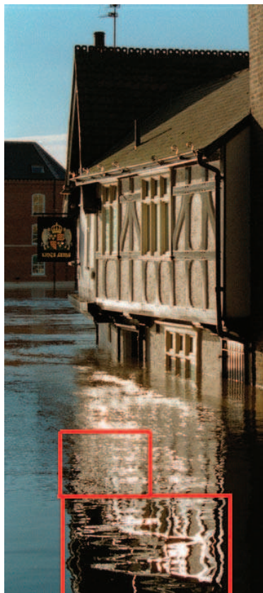
Figure 3. York's Kings Arms pub showing water textures during flood.
