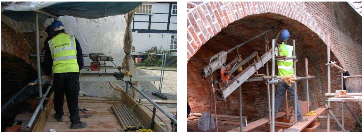
Figure 6. Drilling the transverse holes (left) and longitudinal holes (right) in the arch barrel
