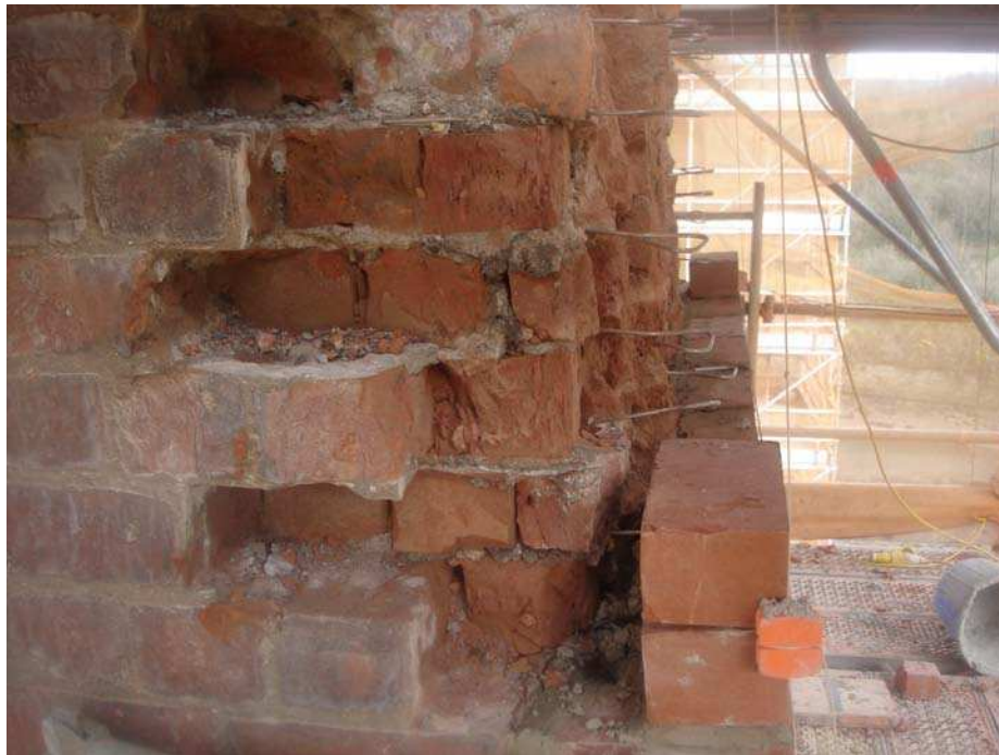
Figure 6. View of the pier rehabilitation works
