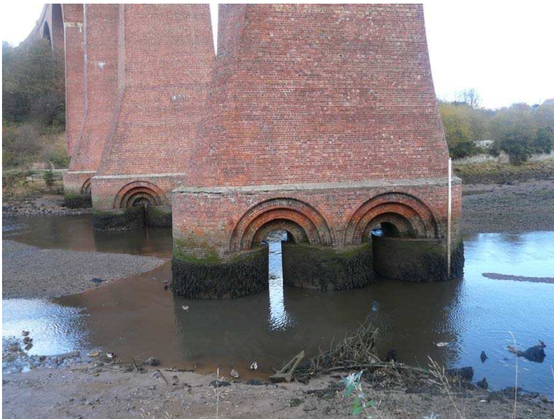
Figure 2. A view of the caissons and arches of the foundations for Pier 5
