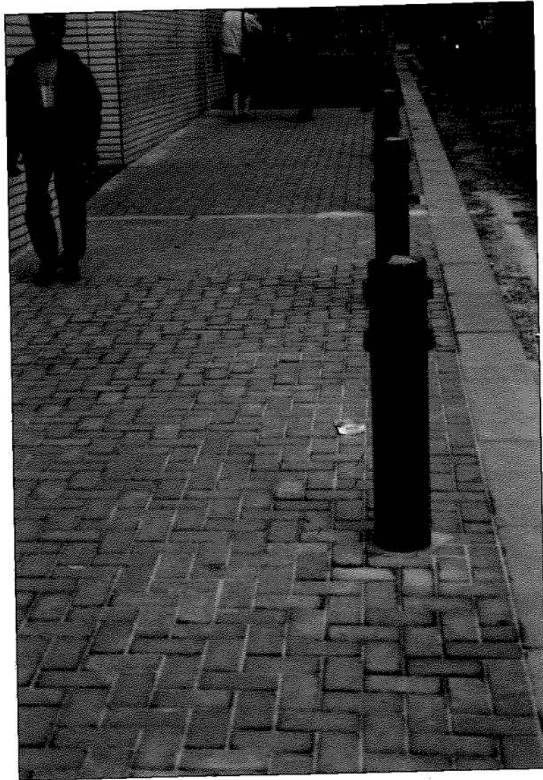
View from Cross Burgess Street
