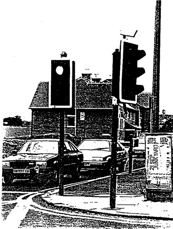
**Figure 3: Microwave Detectors on Existing Traffic Signal**
