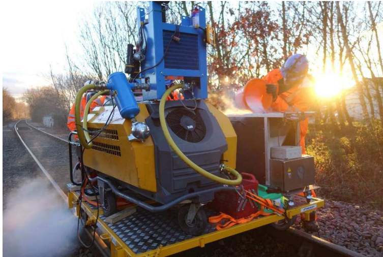
Figure 2. The track trolley mounted equipment in use on a low traffic freight line in South Yorkshire
