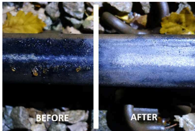
Figure 3. A photograph showing where cryogenic cleaning of the “blackened leaf layer” has stopped
