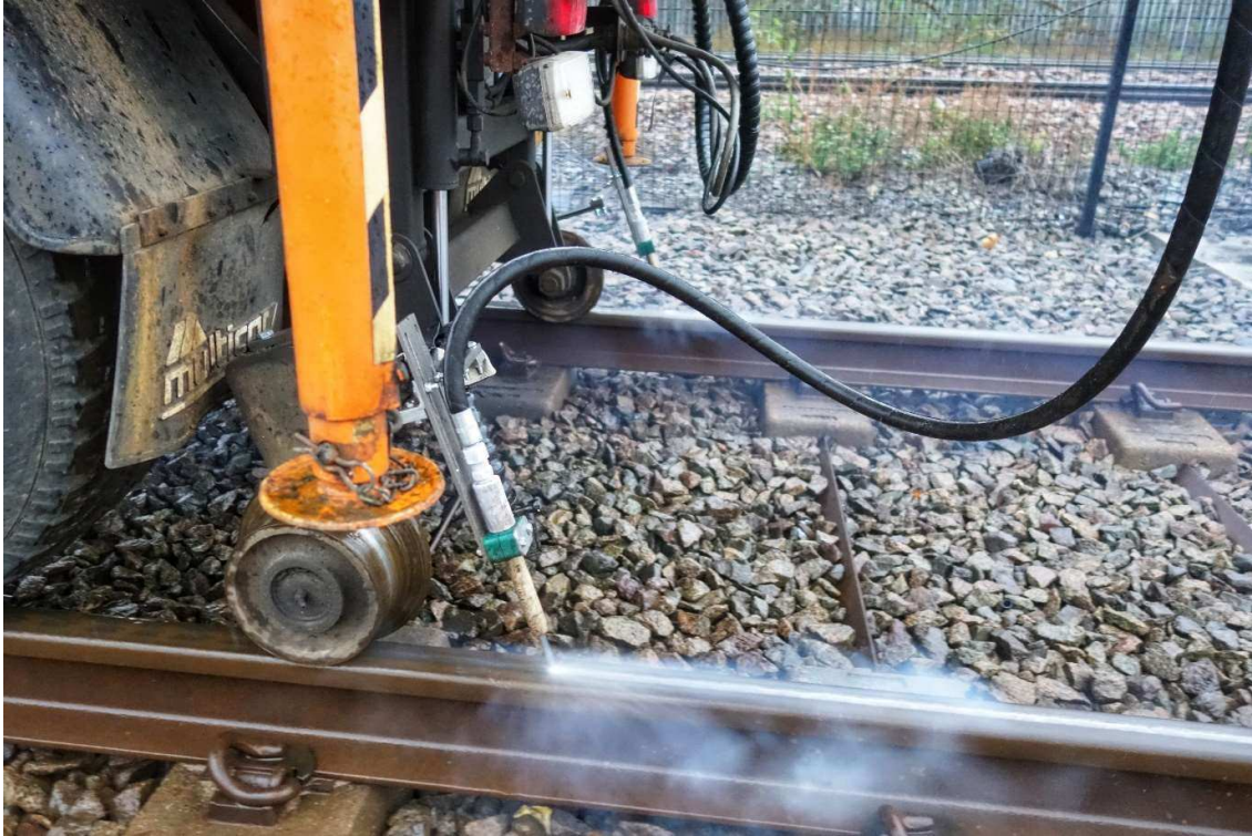
Figure 4. The Cryogenic Cleaning system mounted on the RRV Multicar at Sheffield Supertram Depot, cleaning heavily oxidised track
